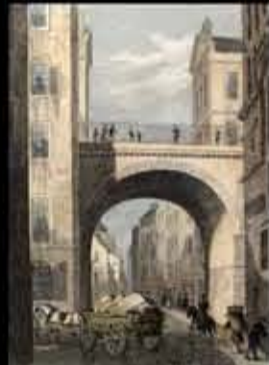
Top - Adam's South Bridge flying over the Cowgate Below - Telford's Dean Bridge over the Water of Leith
