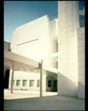
High Museum of Art (1983) by Richard Meier feature white enameled steel cladding
